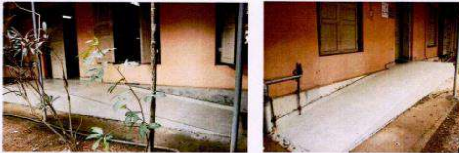
Fig 5 and 6: Ramps to the Electrical workshop area.
