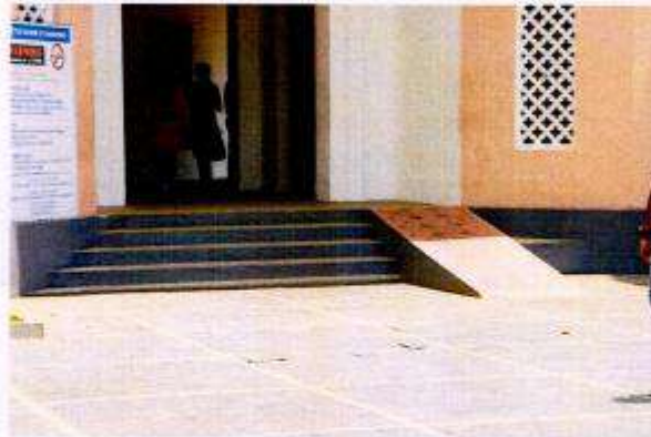
Fig. 1: Ramp provided as access the main entry near the campus gateway.
