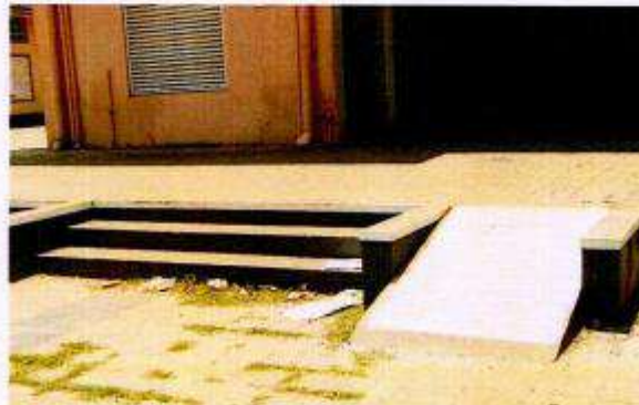
Fig.2: Ramp providing access to the wash room facility.
